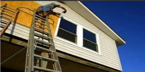
“While you can nail plywood shutters as a last resort just before a storm strikes, repeatedly putting them up and taking them down will damage the area around your windows and doors, and ultimately affect anchorage quality .” (The Weather Channel, 2009)
